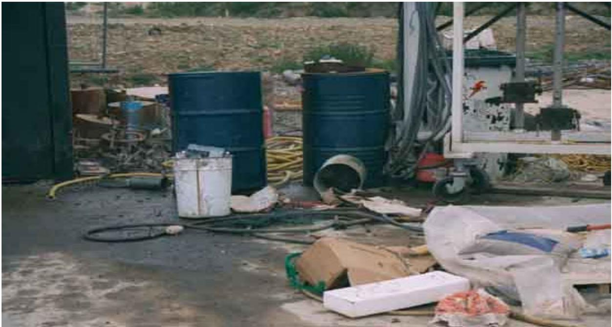
Common faults are Leachate soaking into the ground, no labels on containers and no bunds around the tanks.
