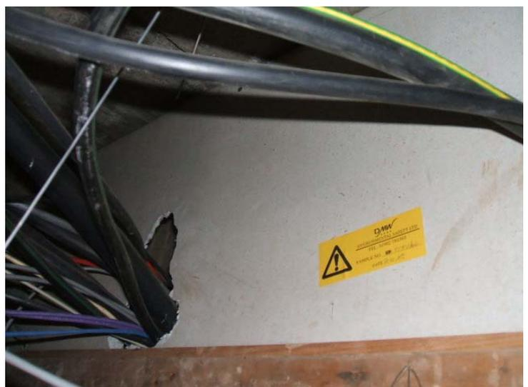
**Damaged Fire Stopping spotted on a DMW Survey. This is dangerous from two standpoints, at least!**
