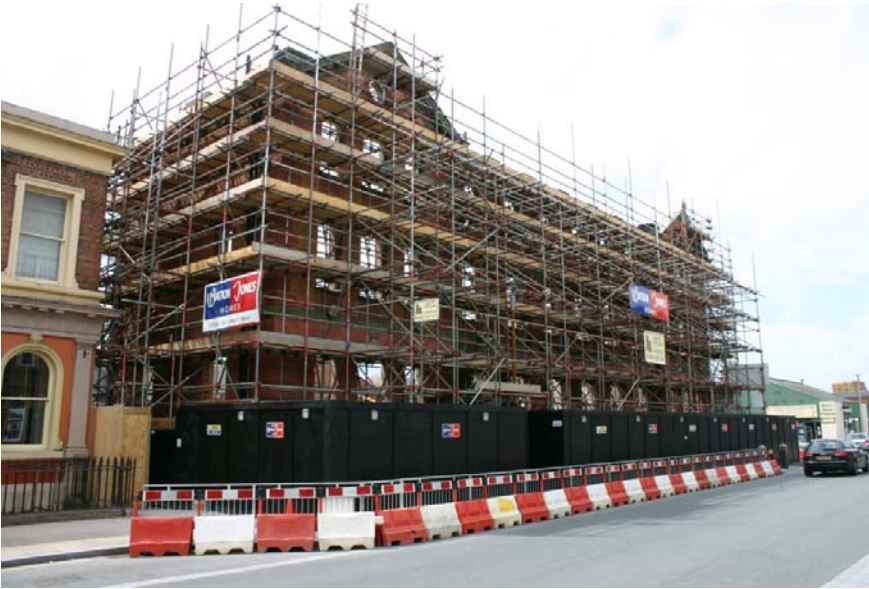
Multiple boarded lifts and working lifts
